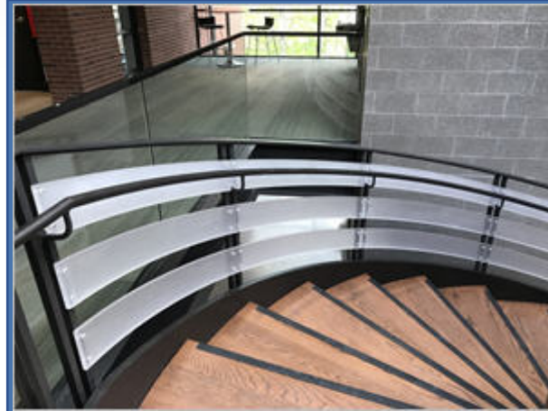
Architectural: Circular Staircase Rails for Eaglebrook School, Deerfield, Massachusetts. Staircase by Charles Wiemeyer.
